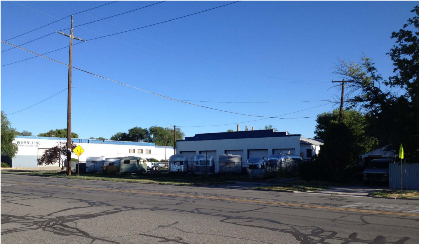
Northwest View of Subject Property from 300 South
