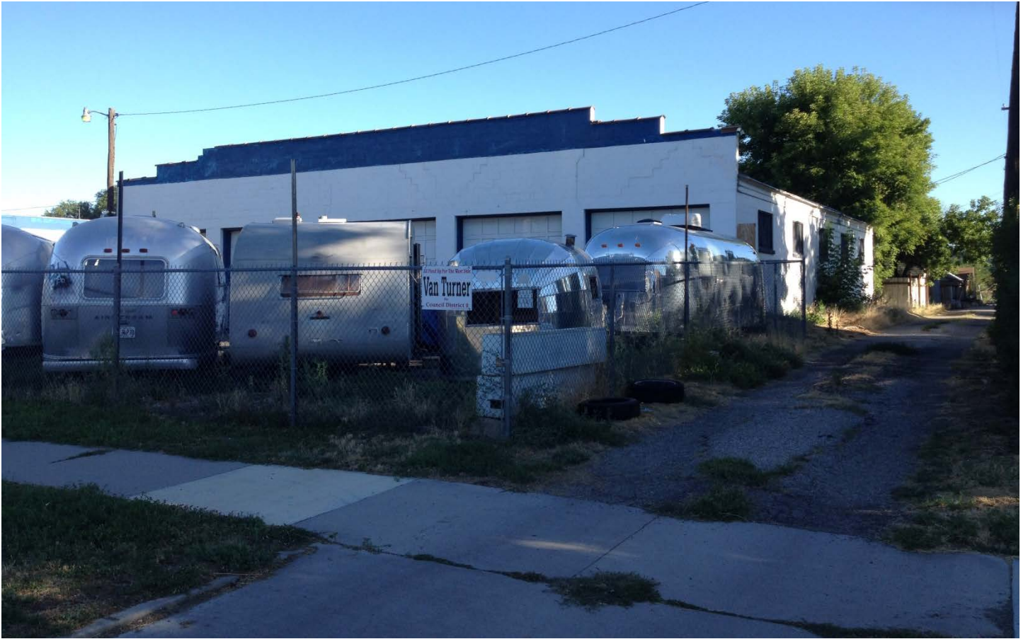
Northward View of Subject Property and Abutting Alley
